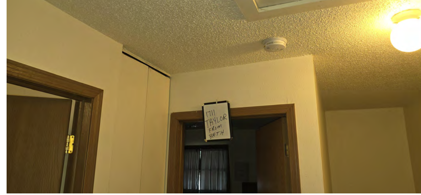
4 2ND FLOOR SITE PHOTO NTS
